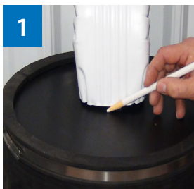
1 Trace downspout on connector
